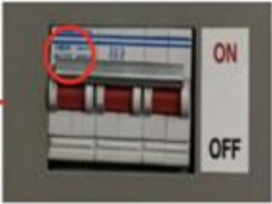
Main Switch Disconnector
